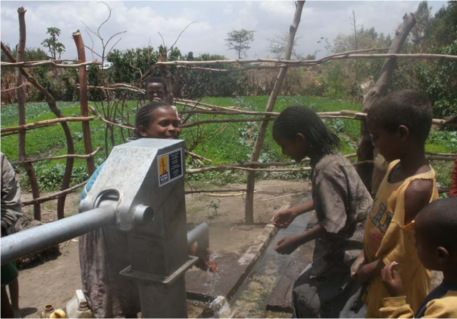
Completed water project and community members gathering to collect clean, safe drinking water.
