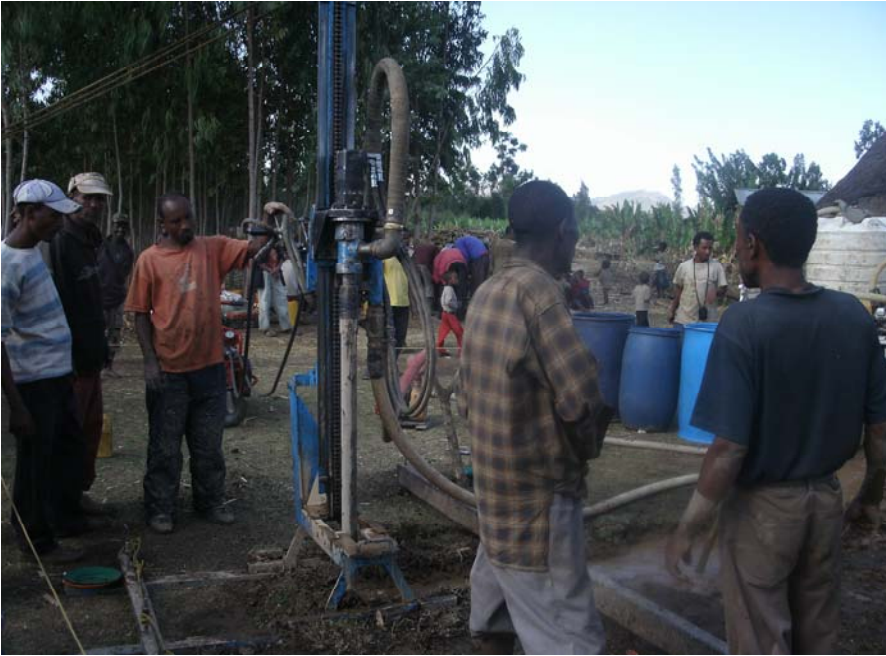
Project in process.
